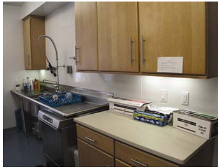
Our new "dishwashing center," complete with a three-compartment sink and commercial dishwasher.
